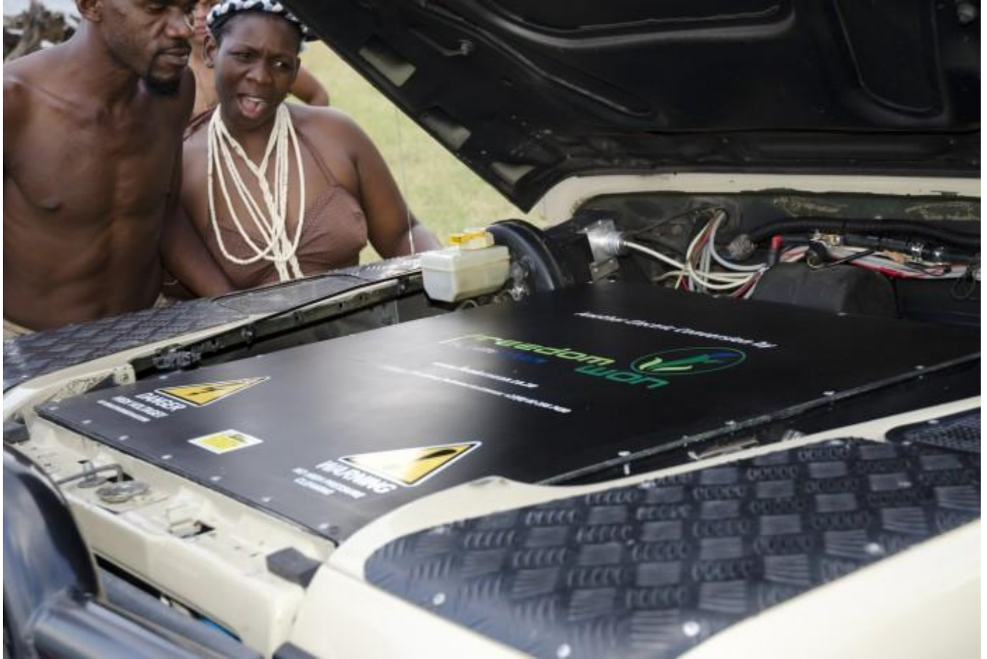
The lithium battery powered engine
